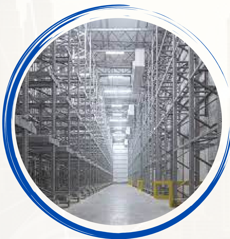
Cold Storage & Warehouse
